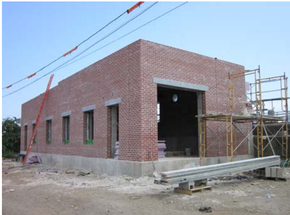
Exterior of the New Aeration Blower Building
