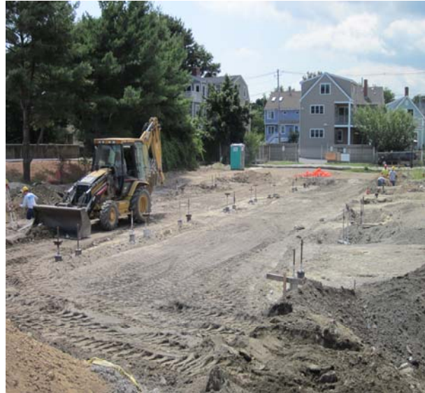
OCL Building Pile Foundation System (view looking towards Water Street)
